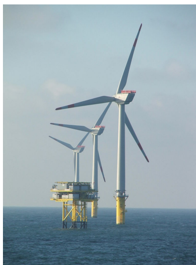
Figure (2.3): Offshore wind farm in the north sea; Source: https://en.wikipedia.org/wiki/Offshore_wind_power
