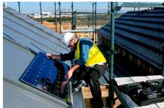
Installing solar panels on the roof of the Village. #
